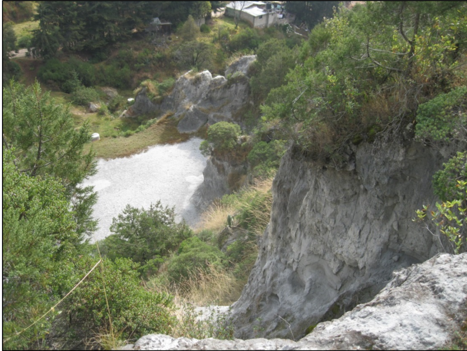
Figure 20.1: Mexico Mine Tailings - Erosional Cuts (near BNO-12)
